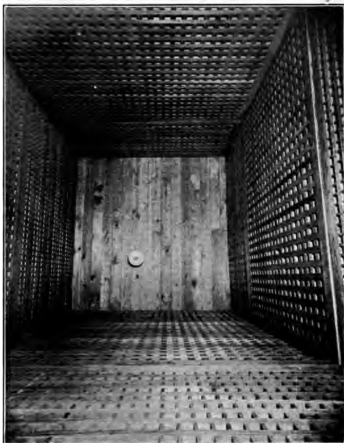
FIG. 10. INTERIOR OF DIFFUSER LOOKING FROM PROPELLER
